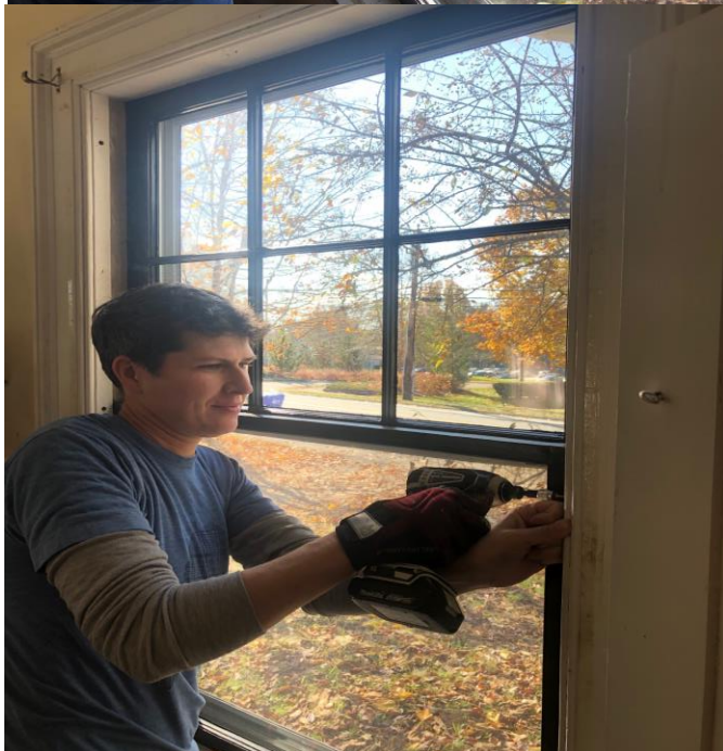
Fitting a newly restored lower sash
